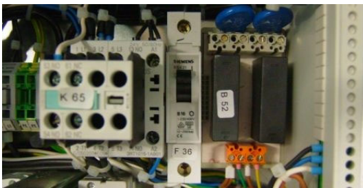
Secondary fuse isolation transformer 1-pole B16A
