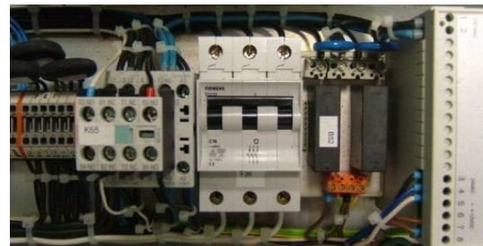
Secondary fuse isolation transformer 3-pole C16A
